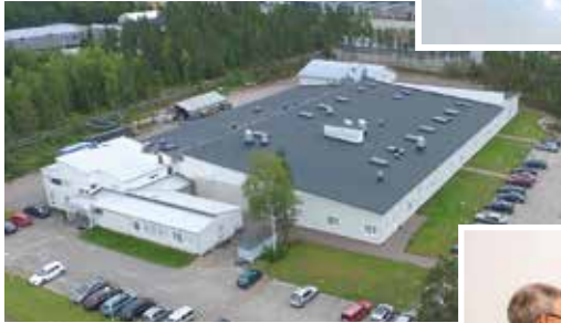
▲ 2016 3rd extension of the Haapavesi facility completed.
